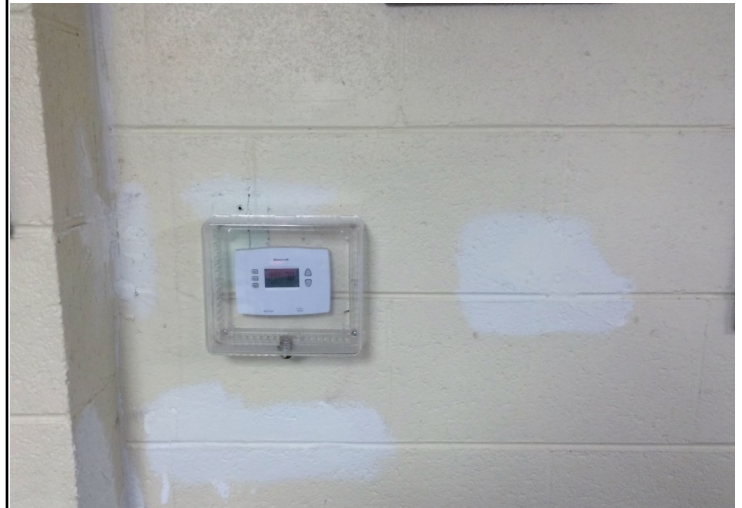
Walls are prepped and ready to be painted
